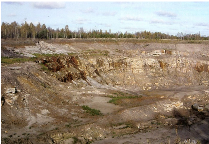
Figure 7 Vishnyakova open pit from which horizontal openings (adits) at the bottom gave access to 12 pegmatite chambers
